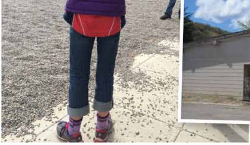
ABOVE: The pea gravel currently in use at MVES playground creates accessibility issues and is a major factor in the wear and tear on district cleaning equipment.
