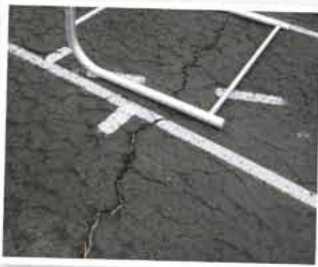
ABOVE/BELOW: Large cracks and deteriorated surfaces put the track and the MVES tennis courts very near the end of servicable use.
