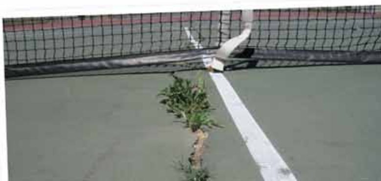
ABOVE/BELOW: Large cracks and deteriorated surfaces put the track and the MVES tennis courts very near the end of servicable use.
