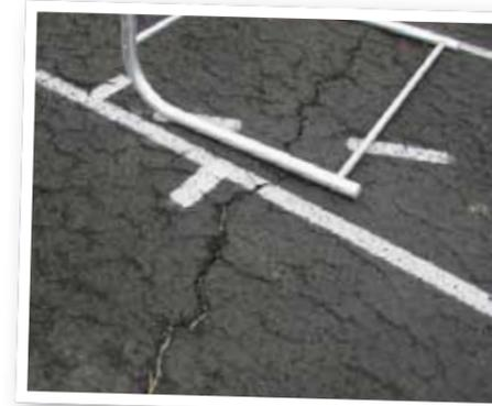
**ABOVE/BELOW:** Large cracks and deteriorated surfaces put the track and the MVES tennis courts very near the end of serviceable use.
